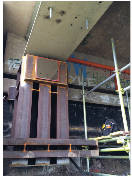
Longitudinal jacking - temporary works
