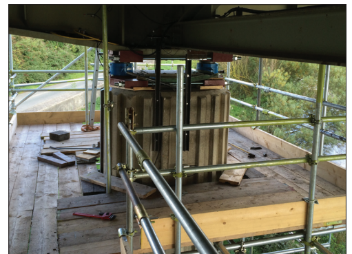
Removal of bearing on pier
