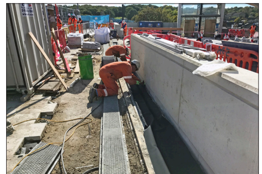
Preparation works for T-Mat expansion joint installation
