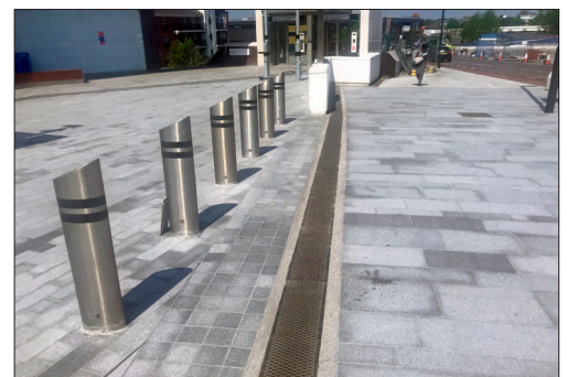
New installed T-Mat 80 expansion joint
