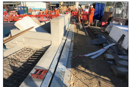
Sub structure steel installed and fixed to concrete prior to T-Mat installation
