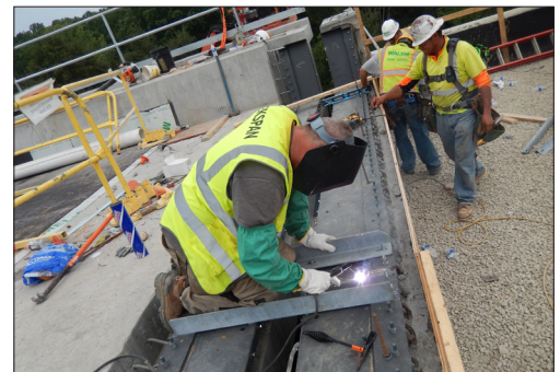
Welding together of steel sub-structure plates
