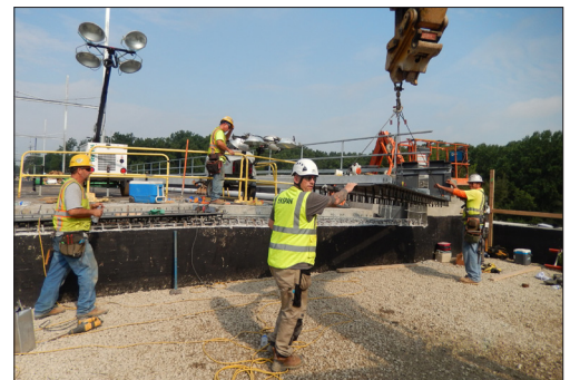
Lifting into position of joint steel sub-structure ready for installation
