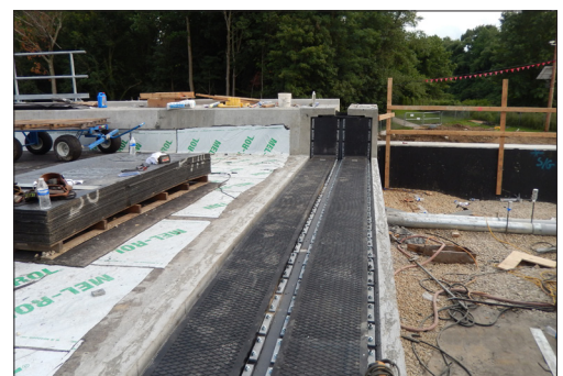
West Abutment - New installed T-Mat 260 expansion joint
