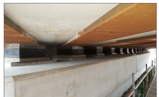
Elastomeric bearings installed
