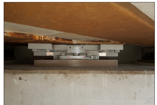
Mechanical bearing installed
