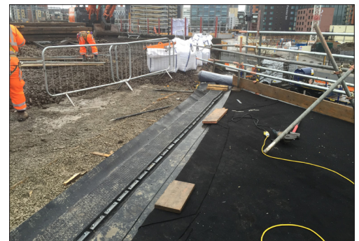
T-Mat 80 expansion joint installed
