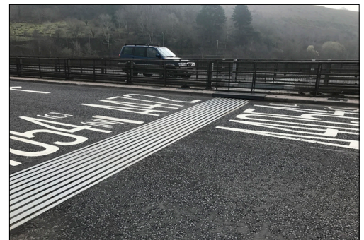
New installed multi-element expansion joint
