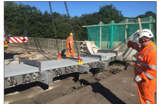
Expansion joint lifted into position
