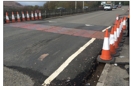
Old expansion joint showing excessive wear
