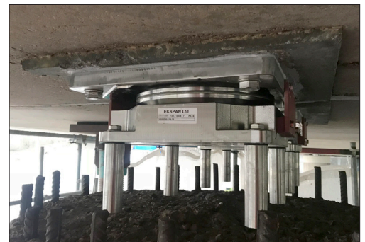
New stainless steel spherical bearing - pre-concrete works
