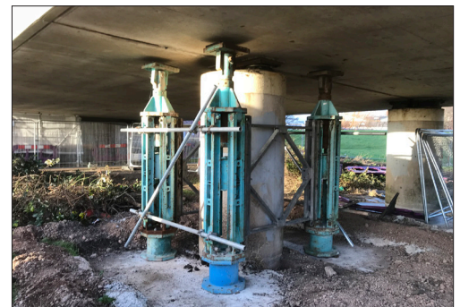
Super props temporarily support the bridge deck during bearing installation
