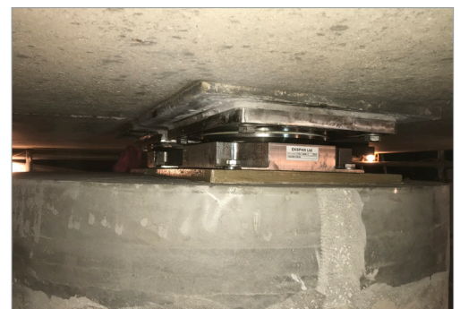
Completed installation of stainless steel spherical bearing
