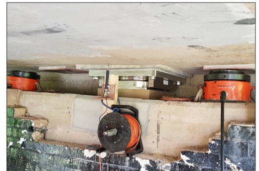
Hydraulic jacks mounted on the bearing shelf prior to bearing installation
