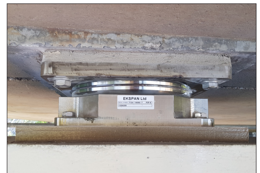
New installed stainless steel spherical bearing
