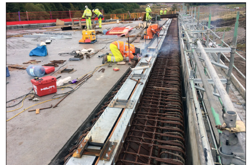
Joint steel rails welded into position for the T-Mat 80 expansion joint to be installed
