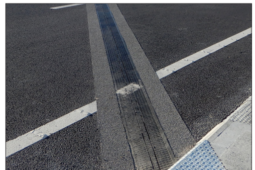
T-Mat 80 expansion joint installed
