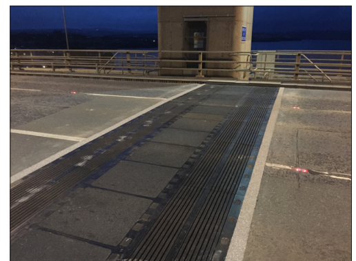
FIP expansion joint installed
