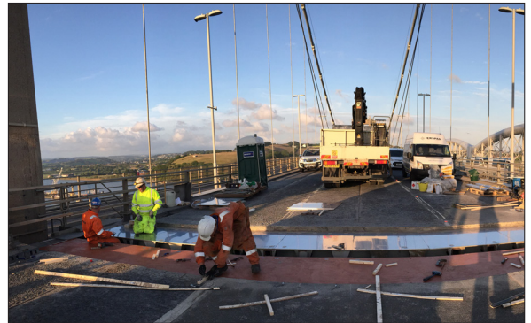
Removal of existing FIP expansion joint plank at the centre of the main bridge deck carriageway
