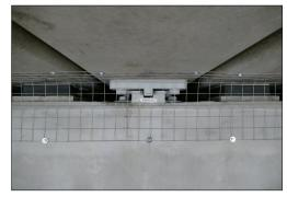
New elastomeric and guide bearings installed complete with pigeon netting
