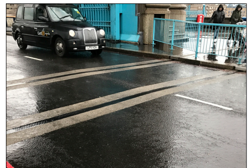
North Approach Span - Installed T-Mat 30 expansion joint across bridge deck
