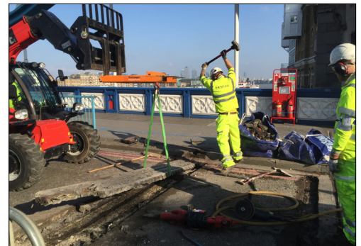
South Approach Span - breaking out of existing Type 6 expansion joint
