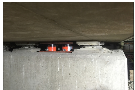
Bearing shelf - localised jacking prior to bearing removal
