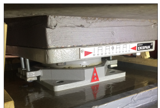
Free bearing installed
