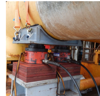
BRIDGE JACKING & BEARING REPLACEMENT
