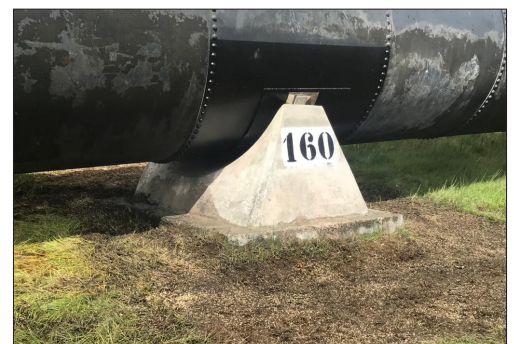
New installed USL Ekspan pipe bearing complete with new concrete bearing plinth.
