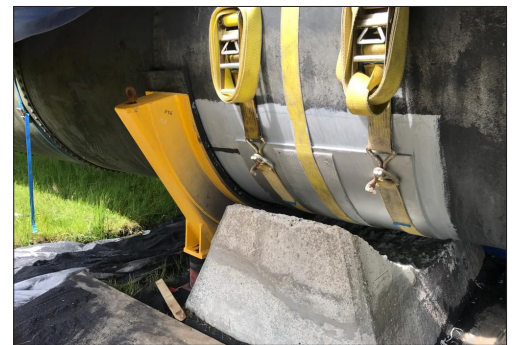
Jacking of pipeline free of existing concrete plinth enabling works for installation of new USL Ekspan pipe bearing.
