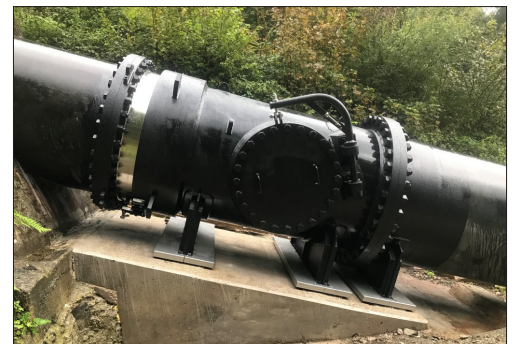
Pipeline Incline - new installed pipe expansion joint section supported on new bearing stools, complete with internal access hatch.
