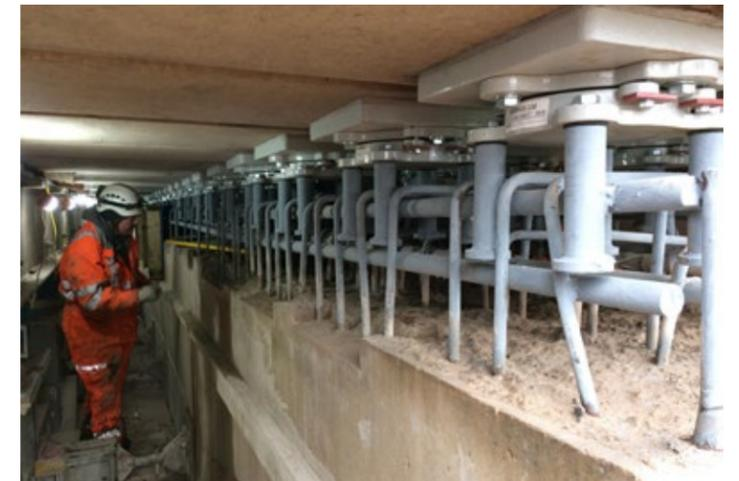
The team overcame challenges with tidal rivers, traffic management restrictions and site logistics to successfully replace all bridge EN-compliant Bearings, a National Highways Mat type replacement Transflex 900 mechanical expansion joint and a Pitchmastic PmB waterproofing system.
